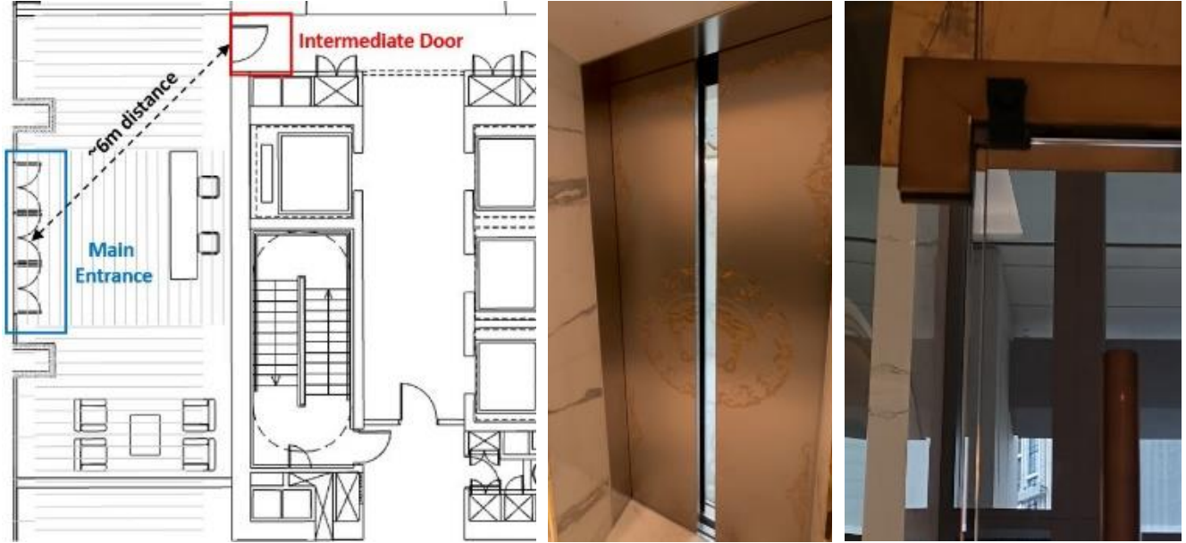
Figure 2. Illustration of ground floor plan (left), gap in lift doors resulting from inability to properly close (middle), and the gap between the intermediate door and its mounting frame (right).
