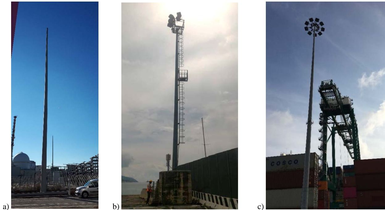
Figure 1. Case studies: 30 m lightning rod (a), 16.6 m lighting tower (b) and 35 m lighting tower (c).
